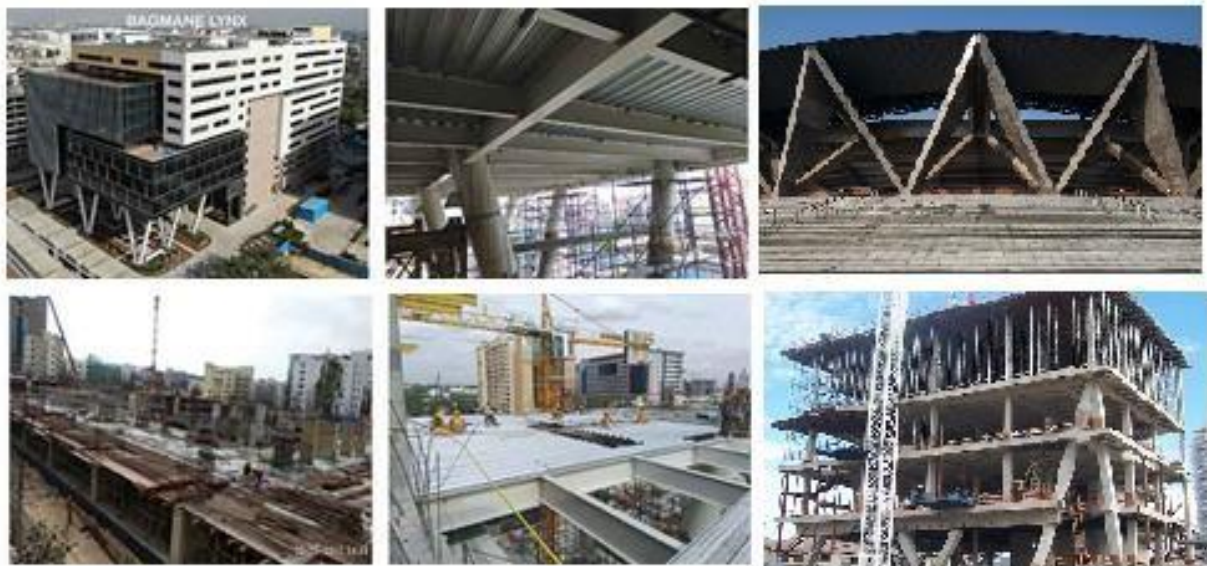
Figure 10: V column construction
