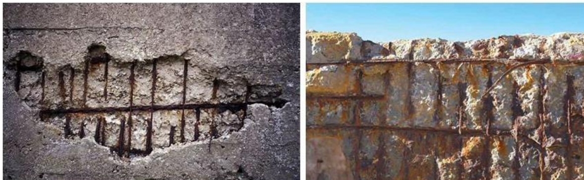
Figure 12: Spalling Concrete
