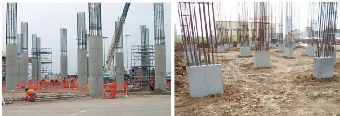
Figure 1: RCC column construction
