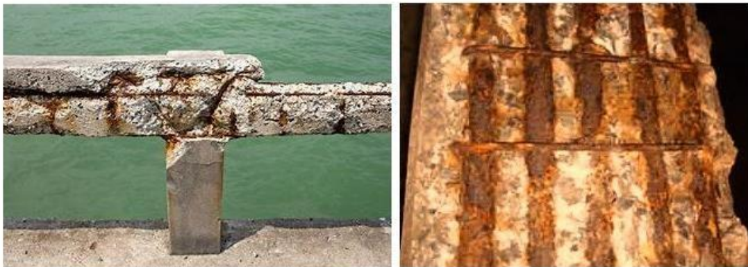
Figure 14: Chloride induced corrosion effect
